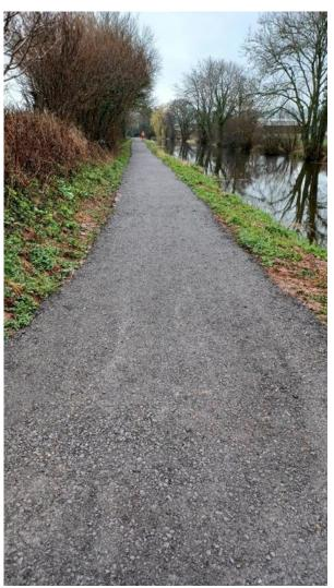
Near Halberton, a section where the path had been worn down to the liner – between Crownhill Bridge and Tiverton Road Bridge - has been resurfaced as shown above right.
