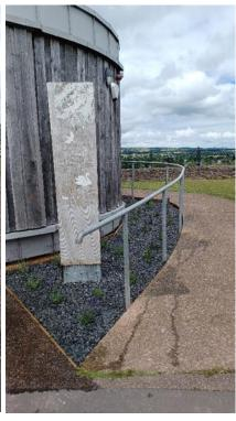
The wooden handrail on the ramp beside the Canal Tea Rooms and Garden has been deteriorating in recent years with some small sections of timber rotting. It was not possible to find a matching handrail and so rather than replacing just the rotted section, the Canal Ranger Service had to replace to whole 40m length.
