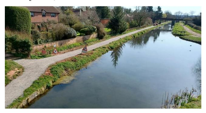
In all cases the path was scraped out at the edges by an excavator and then surfaced to a width of 1.8m and to a depth of 10cm with 20mm limestone scalpings. These were spread evenly and then rolled to compact them.
